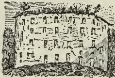
Wall at Zayi.
